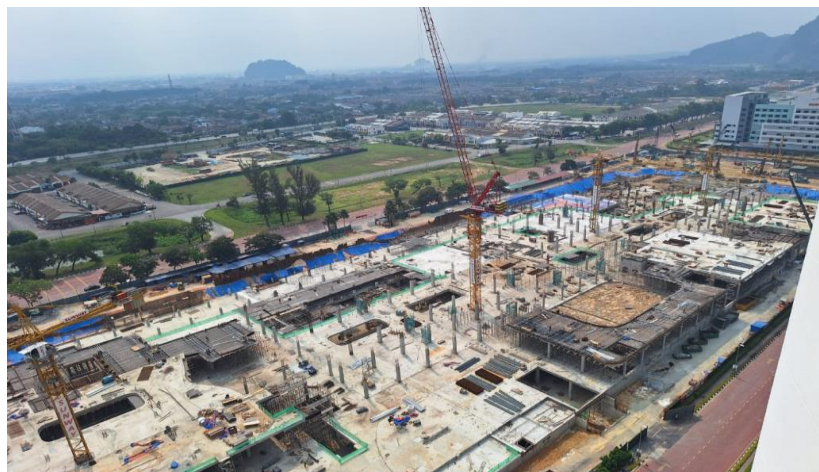
Figure 1: Progress at SCIM's site in Ipoh in July
